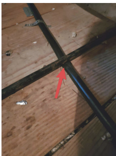
Pinched secondary drain line
