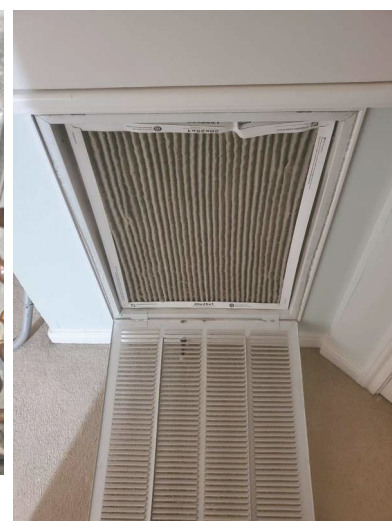
Hallway air filter size 20×25. Needs replacement
