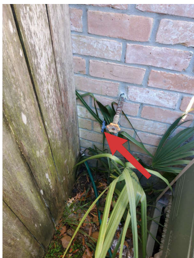
Static Water Pressure Reading: 58 - Home static water pressure was within the acceptable range of 40-80 PSI at the time of this inspection.
