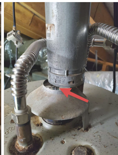
Flue not aligned properly
