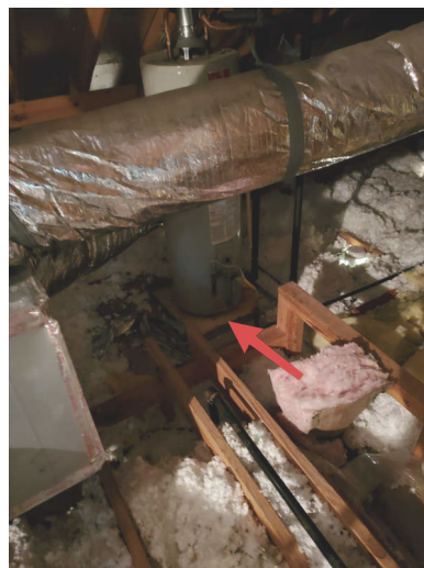
Rusted pan and water heater placed in cramped location
